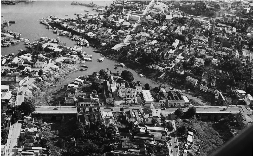
FIG. 4. Aerial photograph (Duarte 2009; view south) of the masonry bridges over Bittencourt (at the left) and Manaus (to the right) Creeks in Manaus (undated image, but approximately 1970). Both bridges were constructed in 1896 to replace the two wooden bridges damaged in the flood of 1892. Both creek channels were backfilled and landscaped in 2006 (Duarte 2009). Note that the water level shown here would conform to the water level of the Rio Negro and the Amazon River for many kilometers up and downstream from Manaus.
