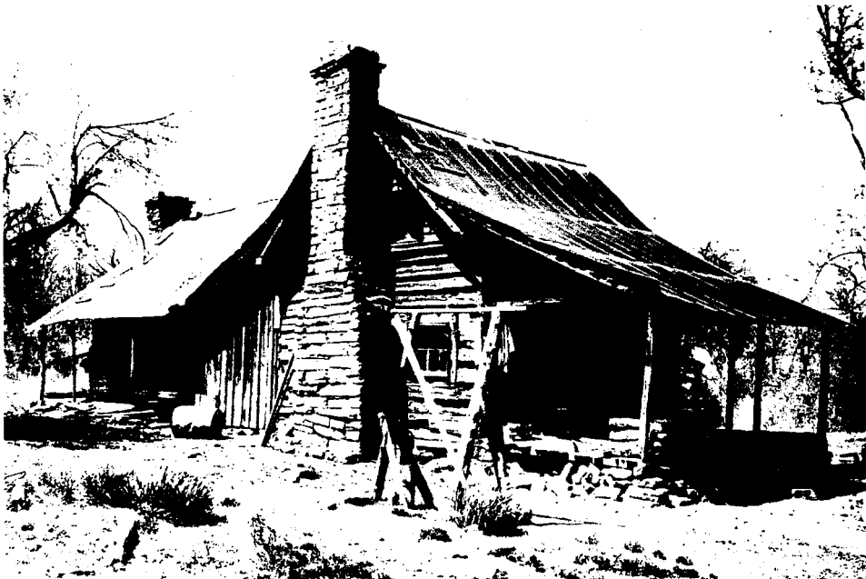
Figure 2. Two white oak log pens of the Jacob King Cabin. Three cutting dates indicate that construction on the front pen began after the growing season of 1888.
